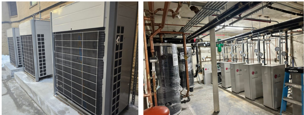
Seneca Avenue: combined heat pump - space heating and DHW
