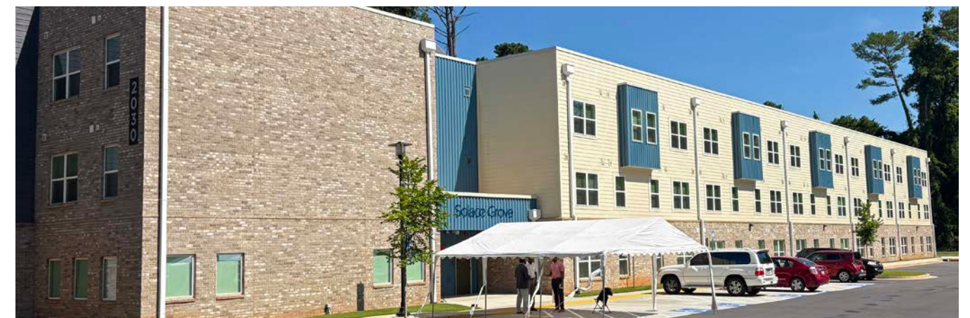
Solace Grove, affordable homes for seniors in Decatur, Georgia, opened its doors in early 2026 with support from Enterprise’s Faith-Based Development Initiative
