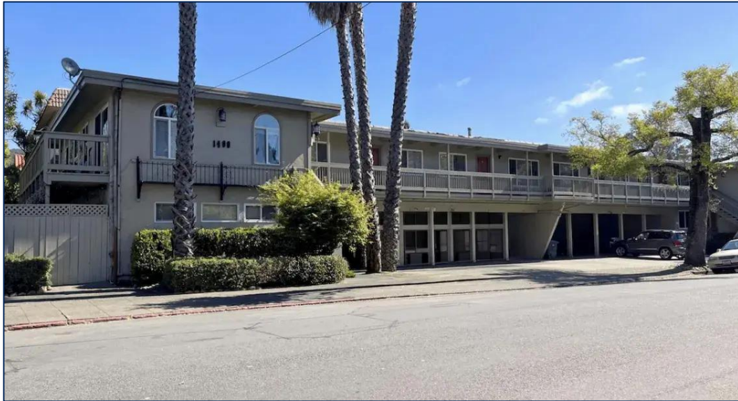
Image source: Canal Alliance's nine-unit acquisition in San Rafael
