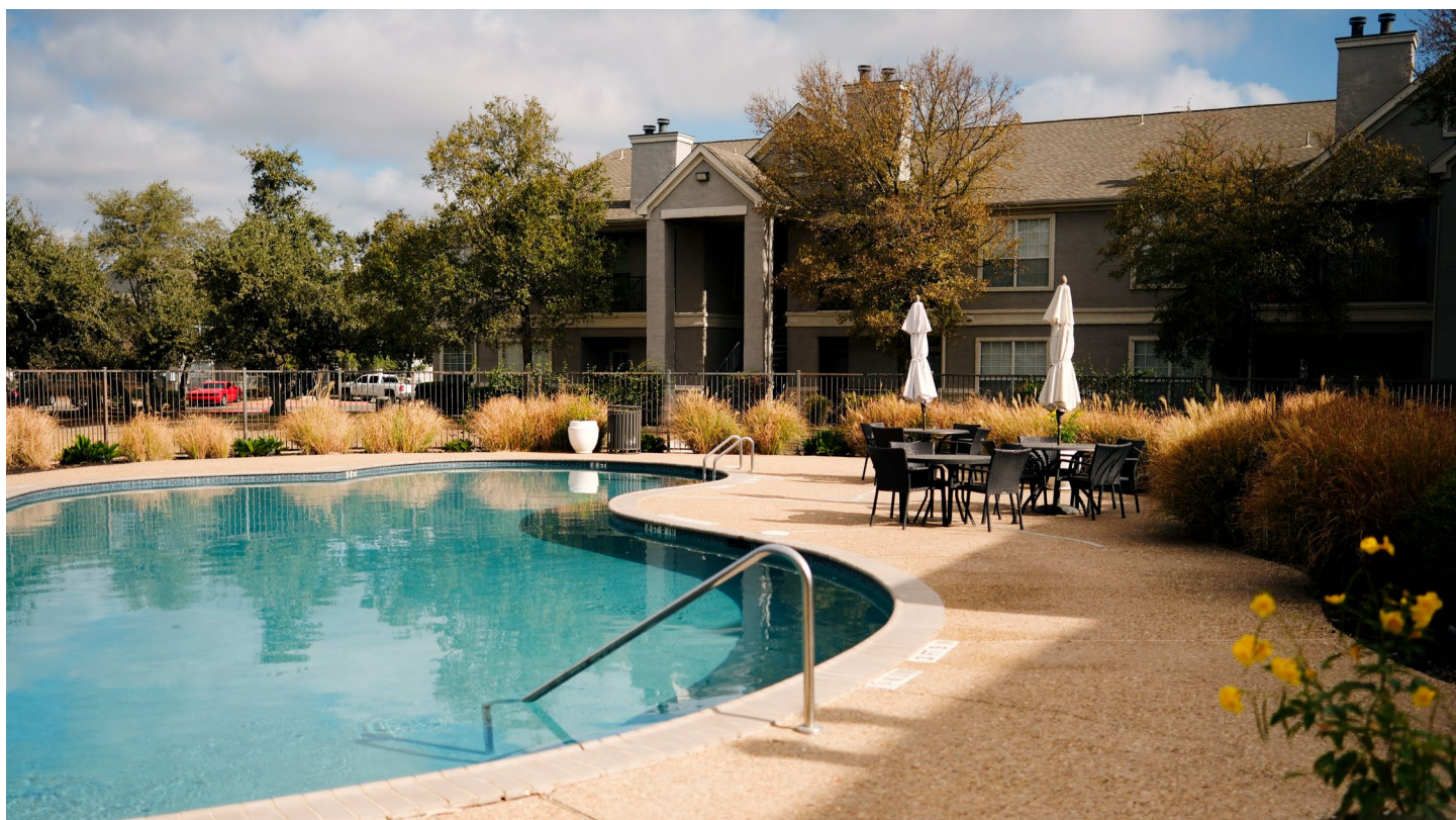
Bridge at Volente in Austin, TX
