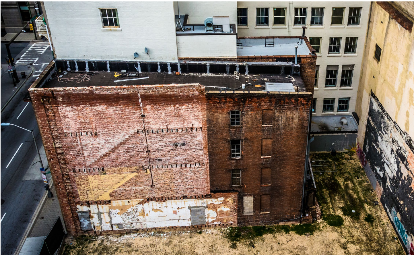
Abandoned building in a U.S. city
