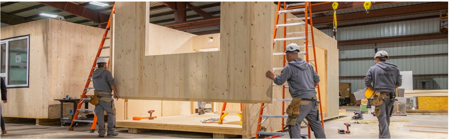
Construction workers build the first modular cross-laminated timber unit in the US, Forterra's ModPro
