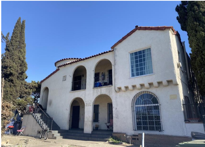
700 Simmons Ave, 11-units, 1930, Unincorporated East LA
