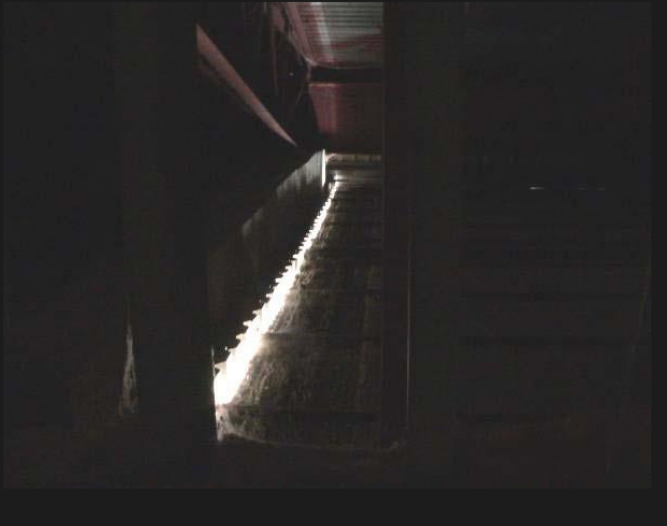
Infiltration Path – Roof/Wall Junction
