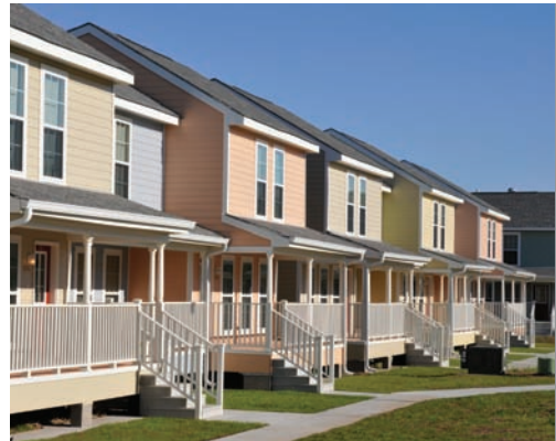
St. Bakhita Apartments is a newly constructed community of 100 green, affordable rental town homes for families in Jefferson Parish, La.
